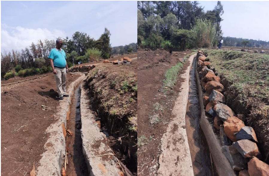
Figure 4: Enebsse irrigation canal
