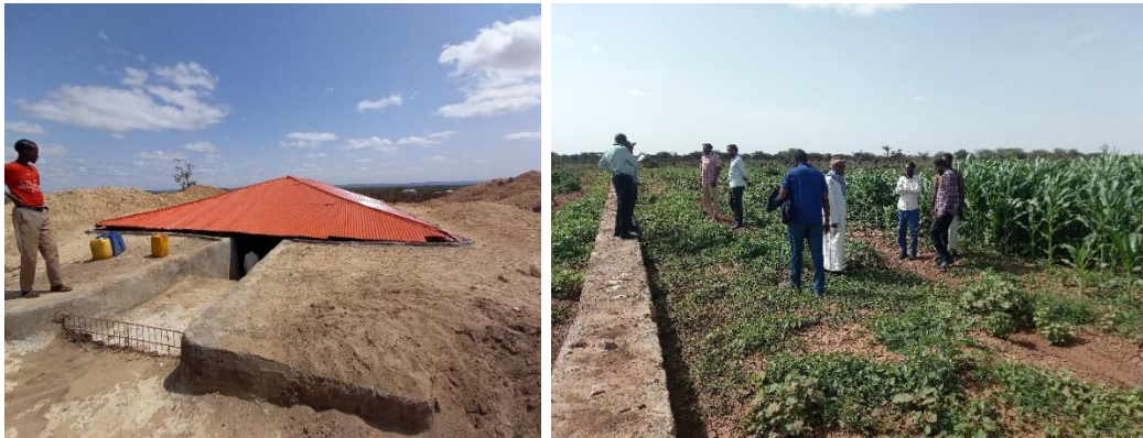
Figure 7: Berkad (Sangomare kebele) and Multipurpose Weir (Helechit Kebele) – Ararso woreda
